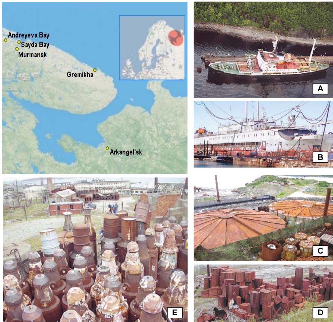
Fig.1 The scope of the SMP: Retired nuclear submarines and vessels: the Floating Maintenance Base Lepse , (A) and a Floating Radiation Control Station, (B); obsolete Dry Storage Facilities for Spent Nuclear Fuel and radioactive waste at Andreyeva Bay (C, D) and corroded Spent Nuclear Fuel containers at Gremikha (E)
